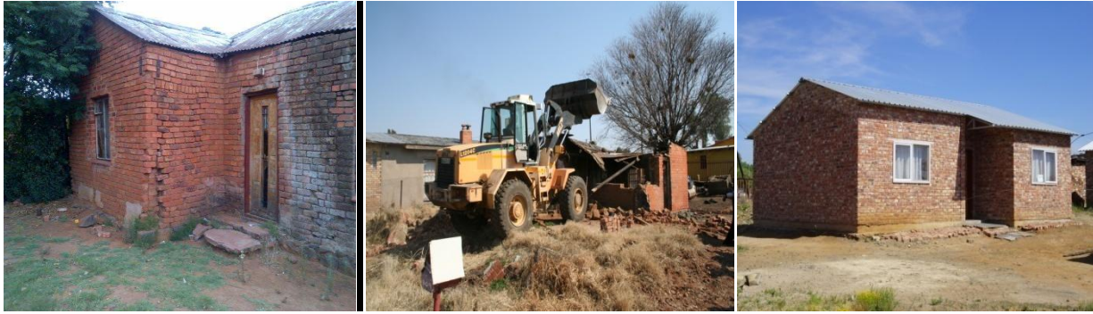
Demolition and reconstruction of better houses, MMM
